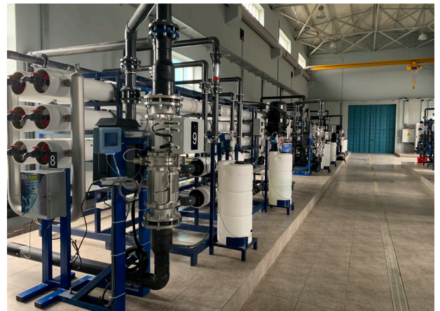
HOD™ UV ensures the delivery of safe drinking water for Agstafa city in Azerbaijan.
